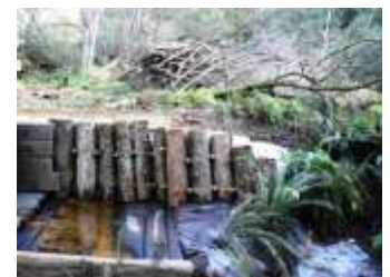
Reusing on-site materials for construction Popes Glen Headwall, Blackheath May 2014
